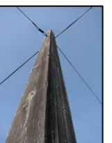
Only two square redwood power poles remain from the days the mill made these poles and provided the power.
