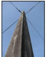
Only two square redwood power poles remain from the days the mill made these poles and provided the power.
